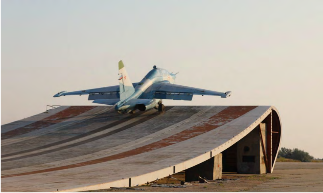
Figure 4.5 Saki Airfield ski-ramp at training range completed. August 30, 2021, https://www.cia.gov/readingroom/docs/CIA-RDP90T00784R000100300001-1.pdf . 109
